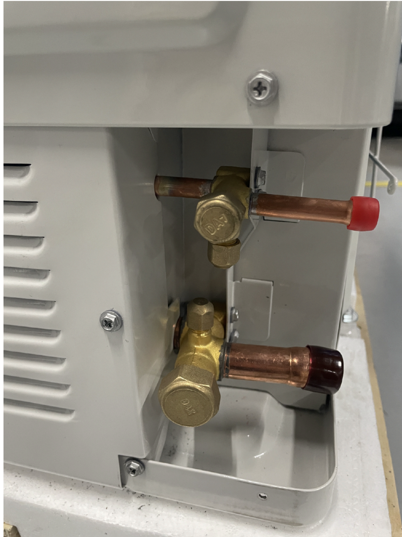
Figure 37: Unit service valves for HH836E2S11
